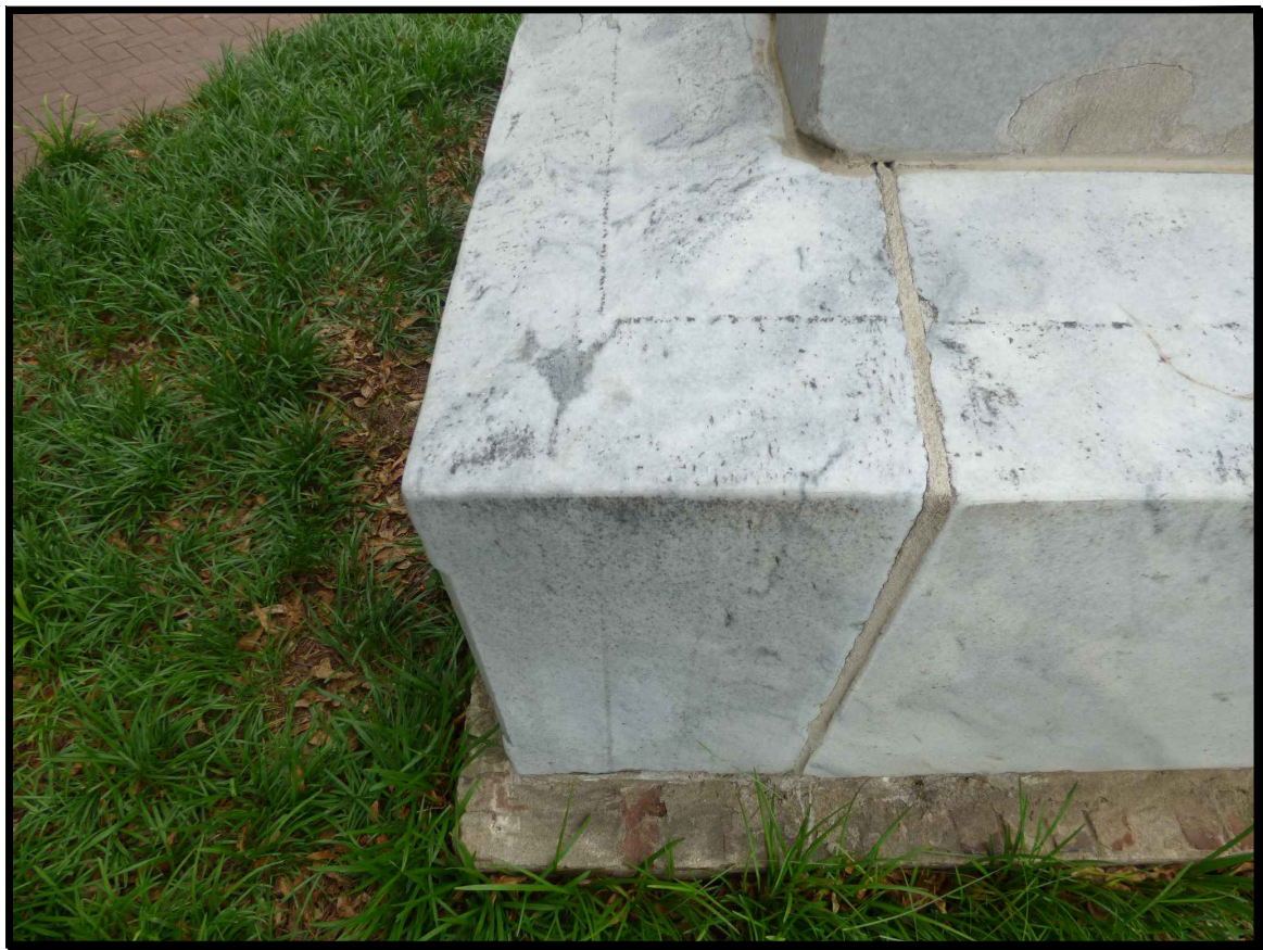
TYPICAL VERTICAL JOINT at 4 PIECE BASE
